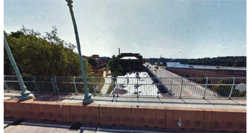
SITE PICTURE 2 – VIEW OVER BUILDING FROM KEY BRIDGE
