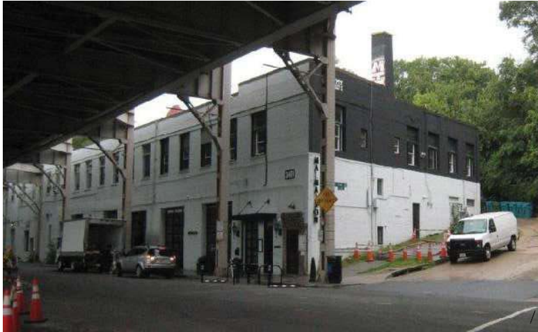
SITE PICTURE 1 – CORNER OF WATER & 34 TH ST, NW
