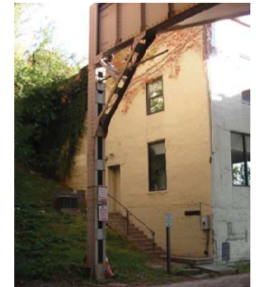
SITE PICTURE 5 – NPS BUILDING
