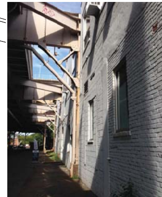
SITE PICTURE 4 – WATER STREET & WHITEHURST FREEWAY STRUCTURE
