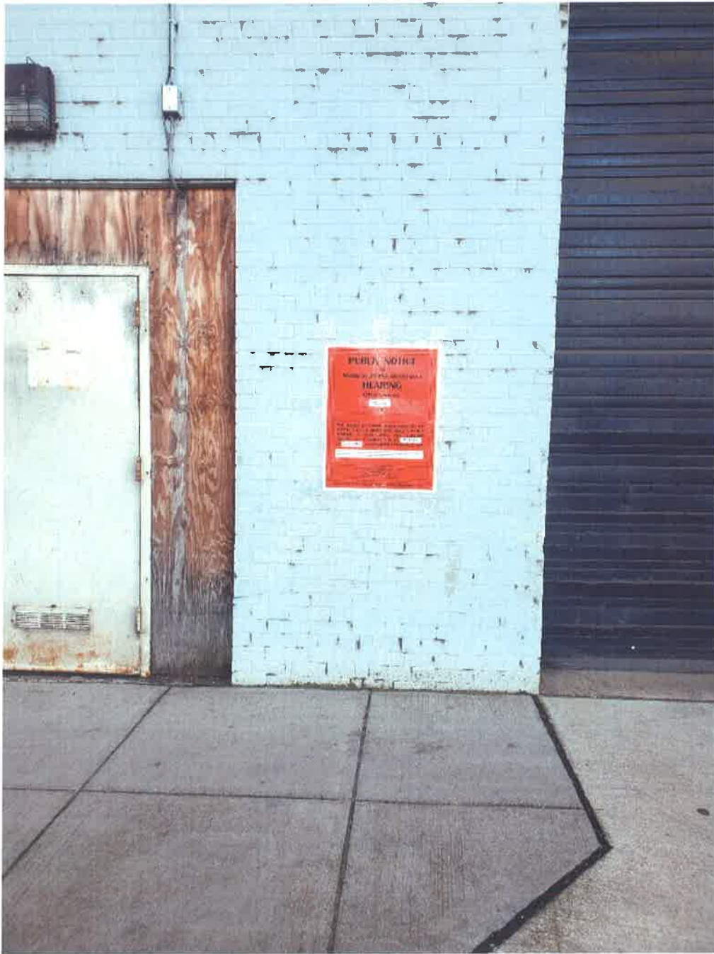
Figure 1 – Sign #1 – Water Street, NW – March 16, 2020
