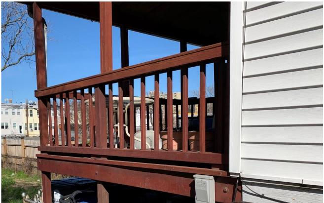
Modified guardrails to be vertical instead of horizontal, ensuring there is no obstruction to the line sight from neighboring decks by allowing ample space between guardrails, as allowed by code.
