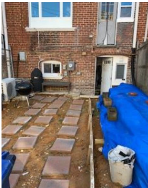
Existing Rear of House
