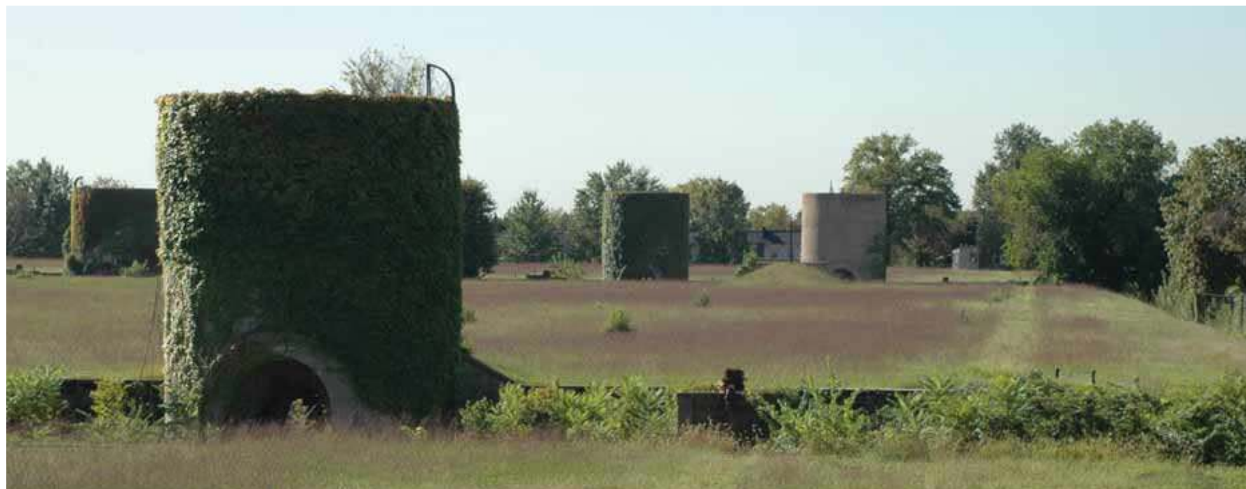
McMillan Site, existing condition
