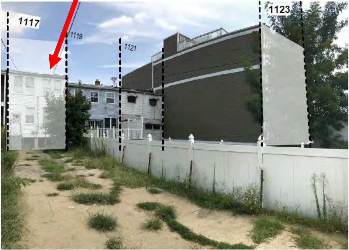
Rear Side View East
