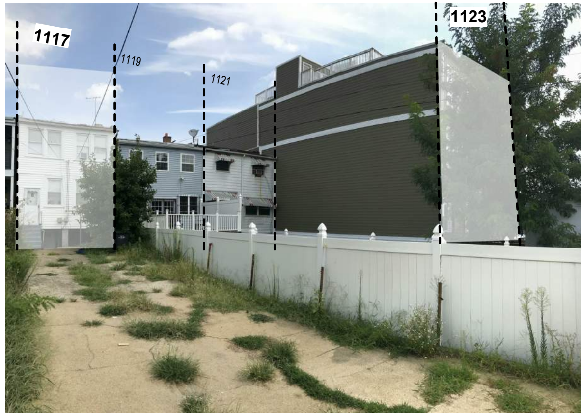
Rear Side View East
