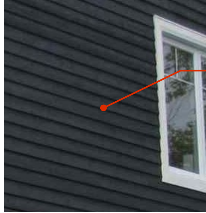
Fiber Cement Lap Siding
