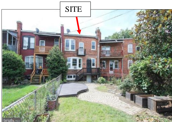
Existing Rear of Houses
