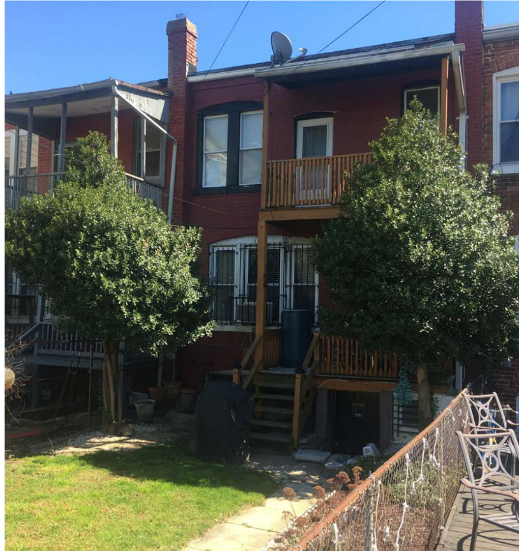
132 Rhode Island Avenue NE Eastern Adjoining Rowhouse
