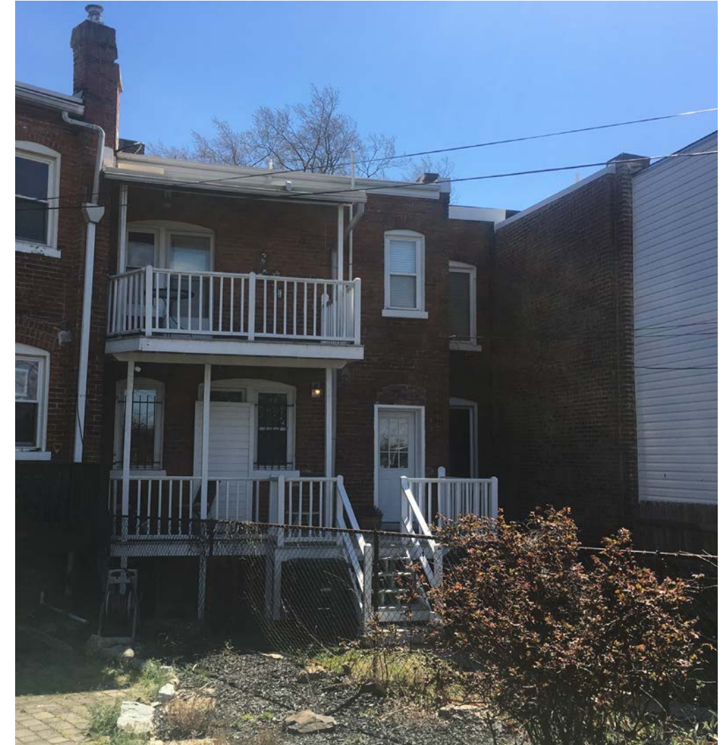
128 Rhode Island Avenue NE Western Adjoining Rowhouse
