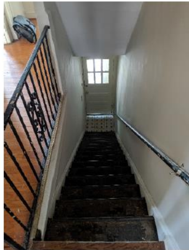
1 (Main Hall – View toward front entrance)
