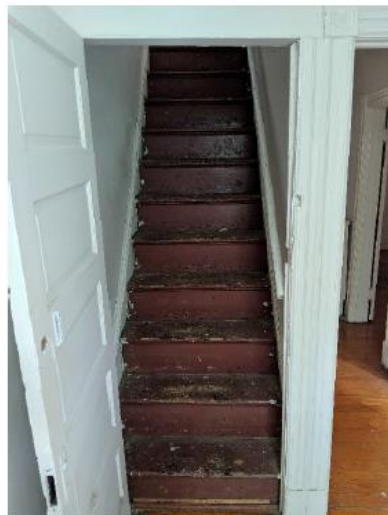
6 (View toward stair to third floor)
