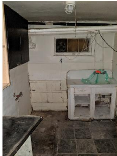
2 (Kitchen – Sink and gas line)
