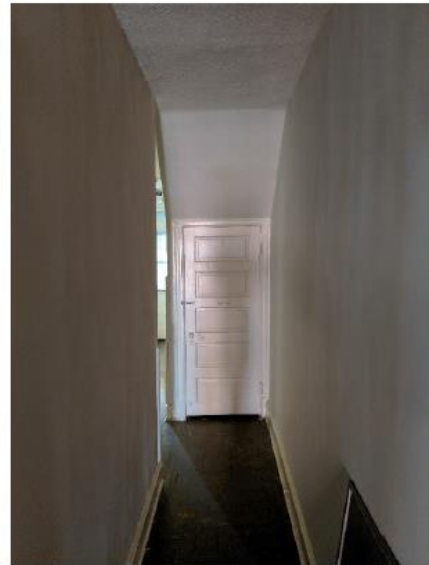
2 (Main Hall – View toward front entrance)
