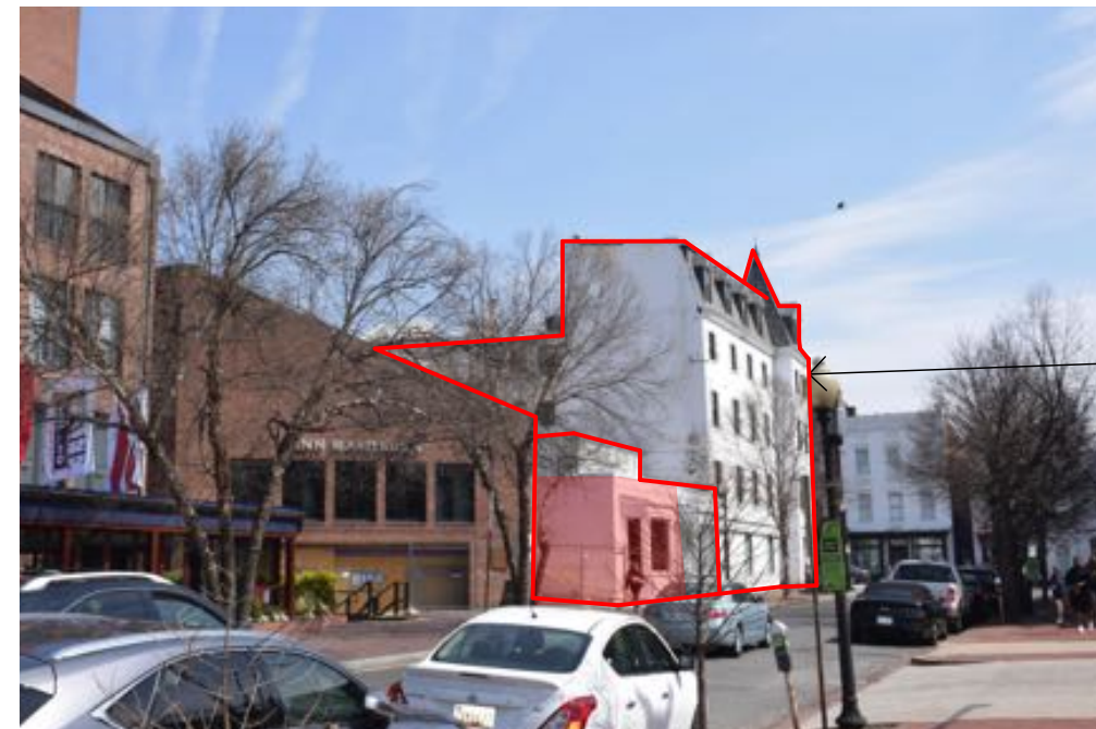
3. View from West, Prospect Street
