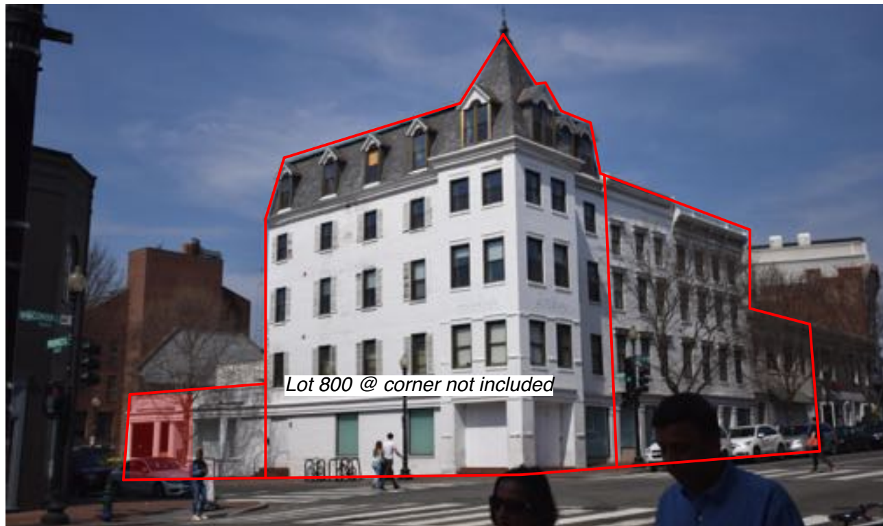
1. View from corner, south east along Wisconsin Ave, Prospect Intersection
