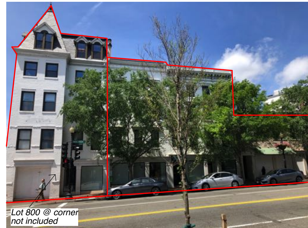
2. View from Wisconsin Ave
