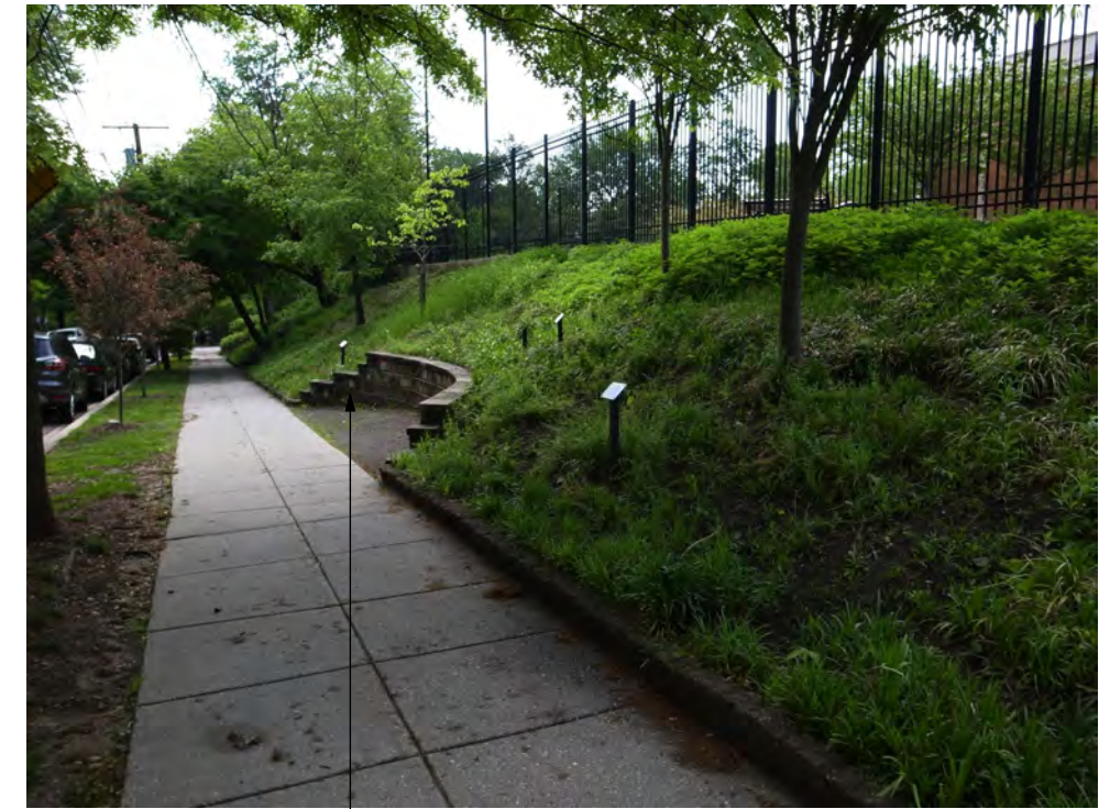
Existing Curved Retaining wall 3' high, typ to be removed
