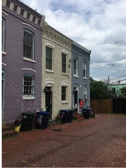
Contextual views of the property and row from the front
