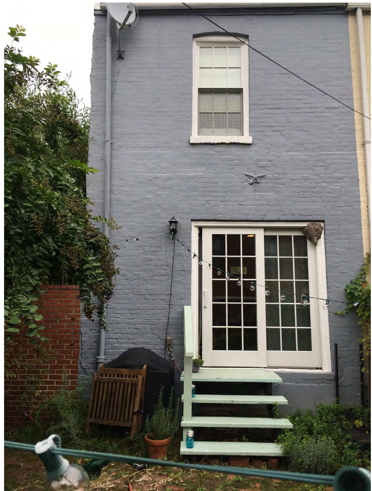
EXISTING REAR FACADE
