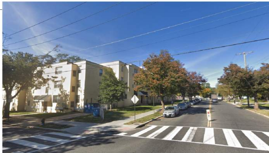
NORTH WEST CORNER OF MONTANA-SARATOGA
