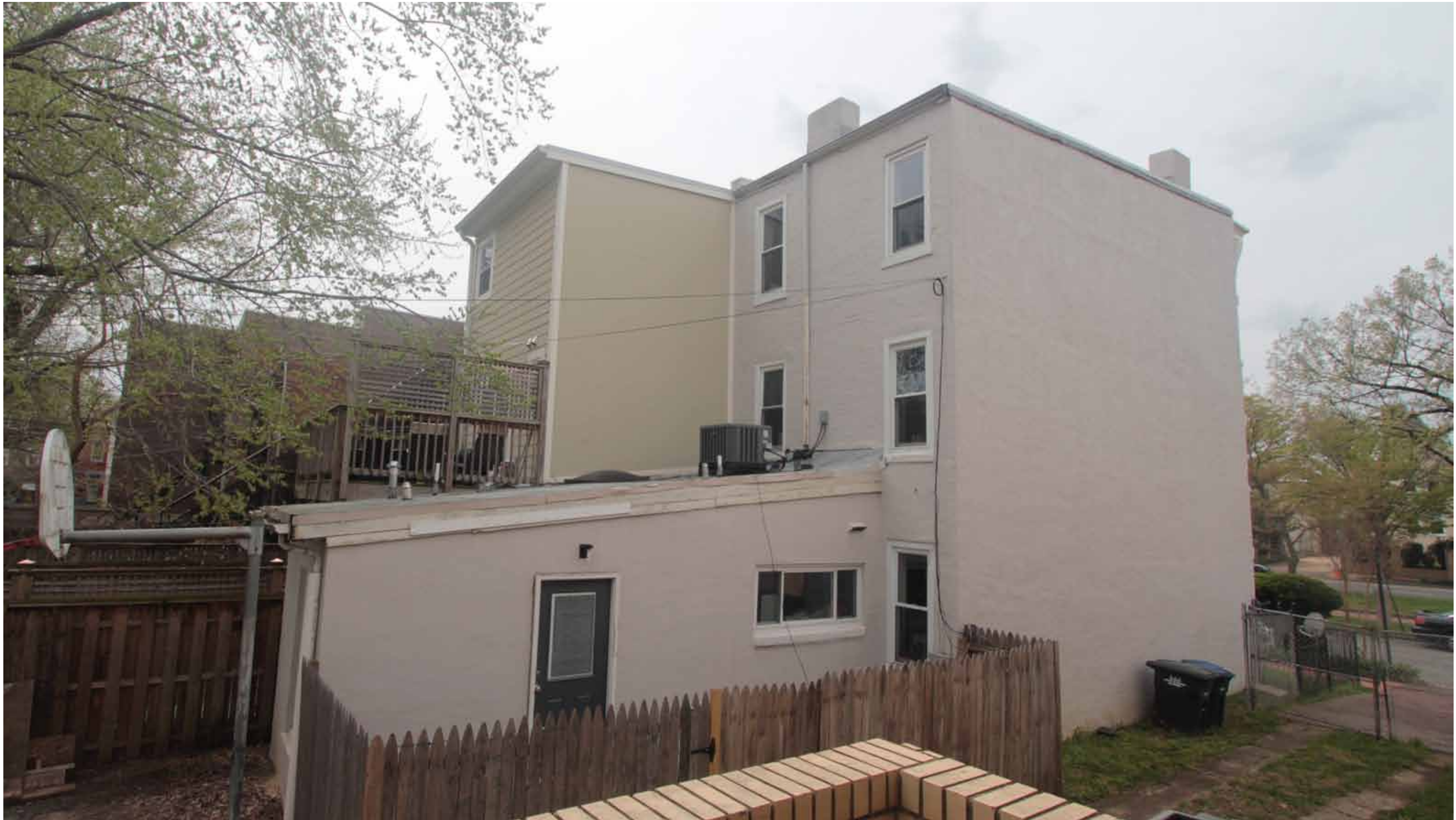
Rear view from south stair
