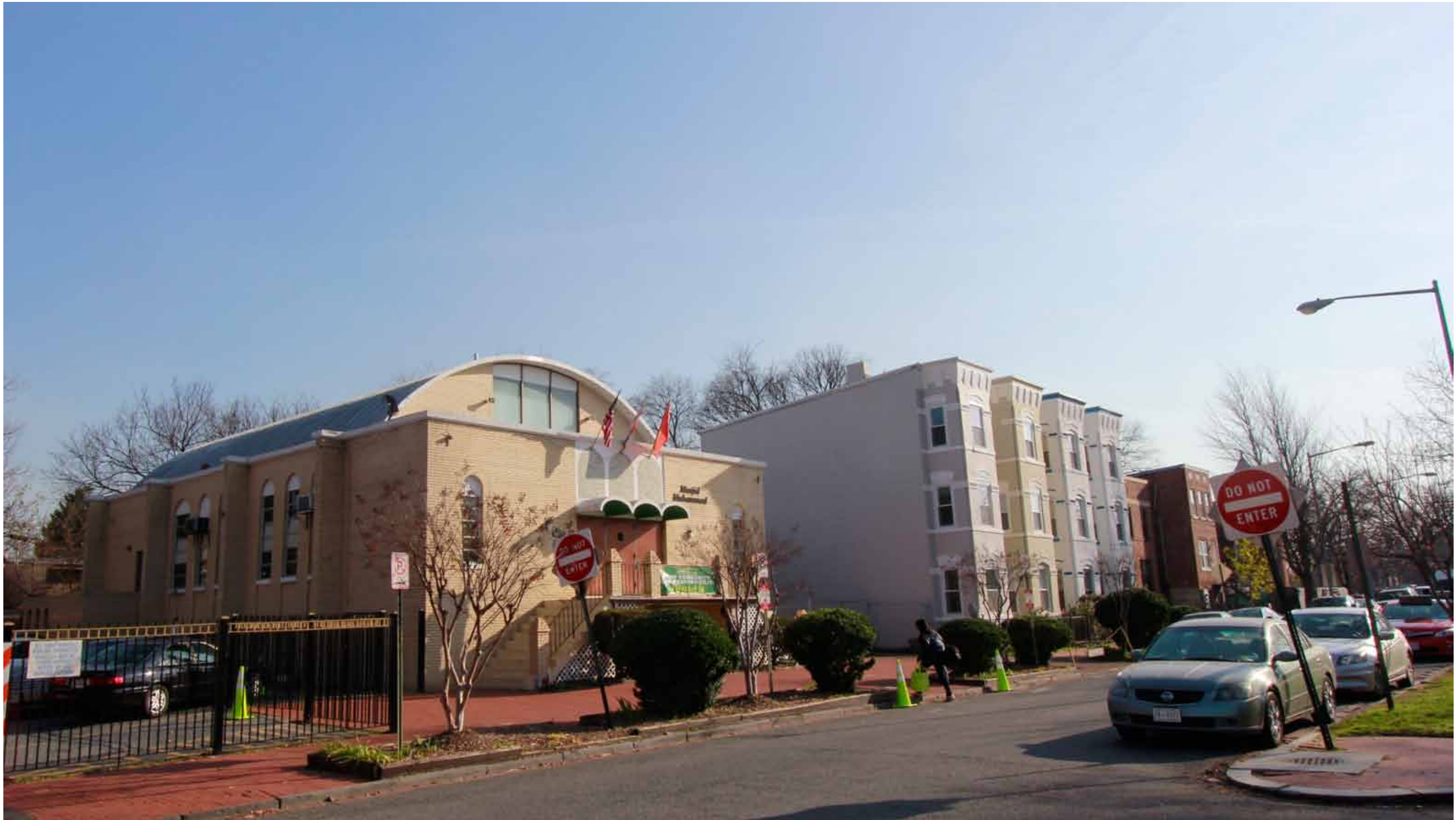
Front view from 4th st
