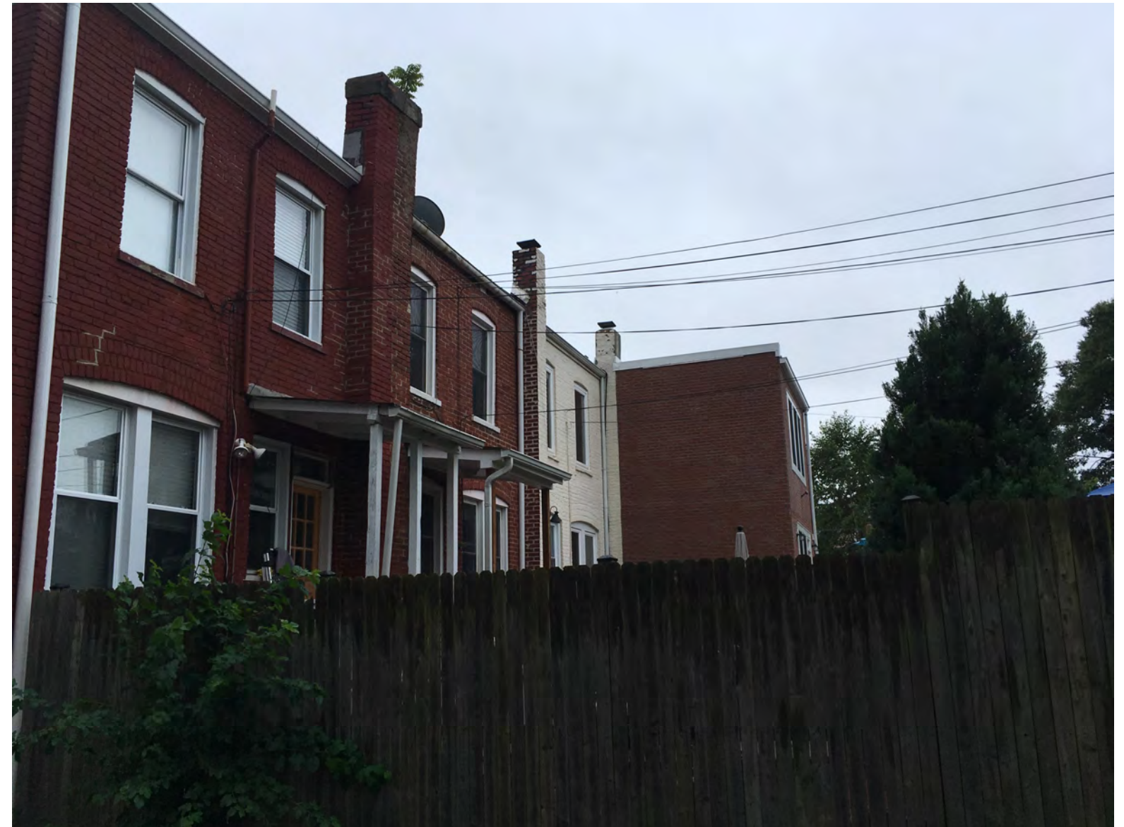
REAR VIEW FROM SIDE ALLEY (LOOKING EAST)
