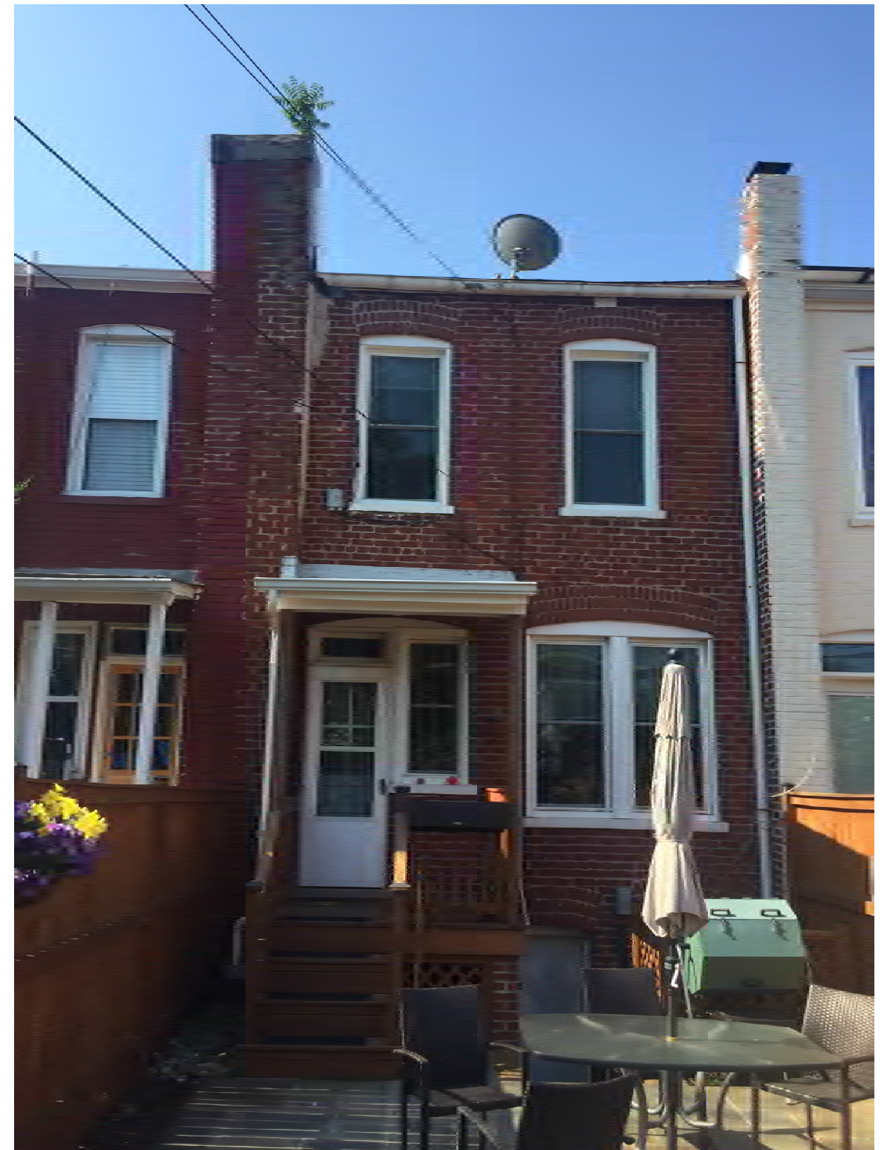
EXISTING REAR FACADE
