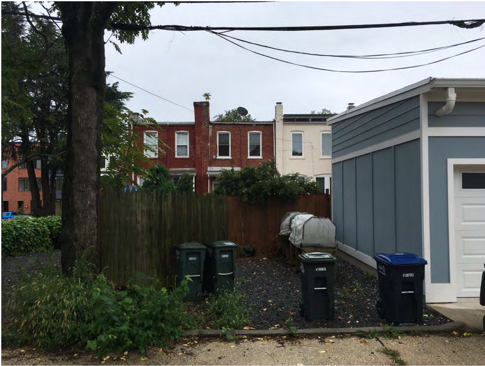
REAR VIEW FROM REAR ALLEY
