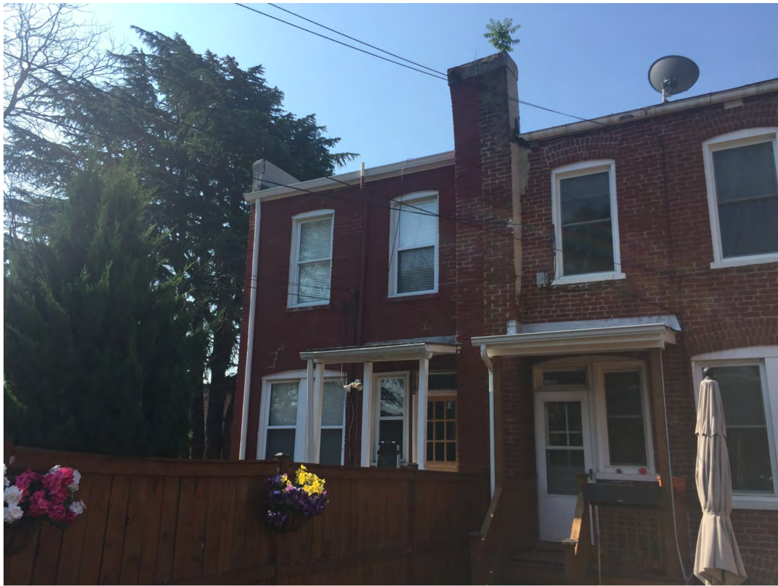
REAR VIEW LOOKING WEST
