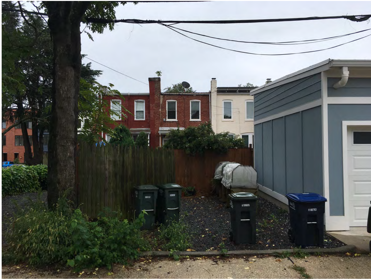
REAR VIEW FROM REAR ALLEY
