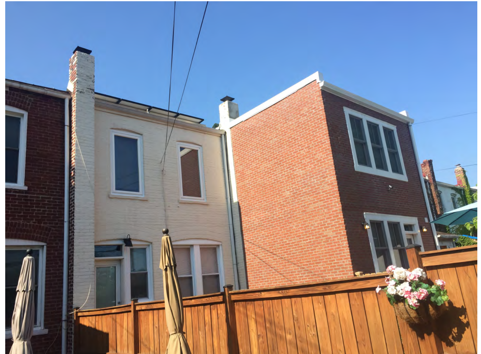
REAR VIEW LOOKING EAST
