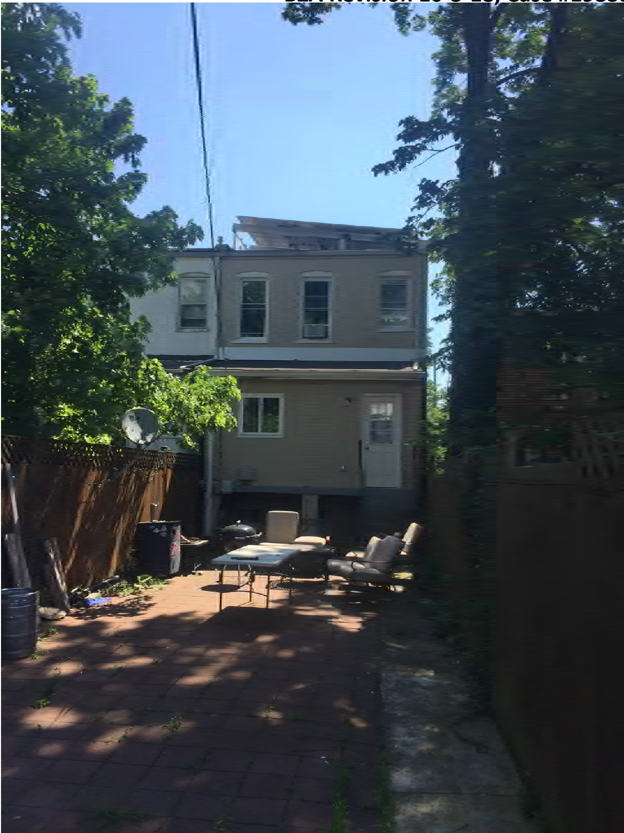
EXISTING REAR YARD
