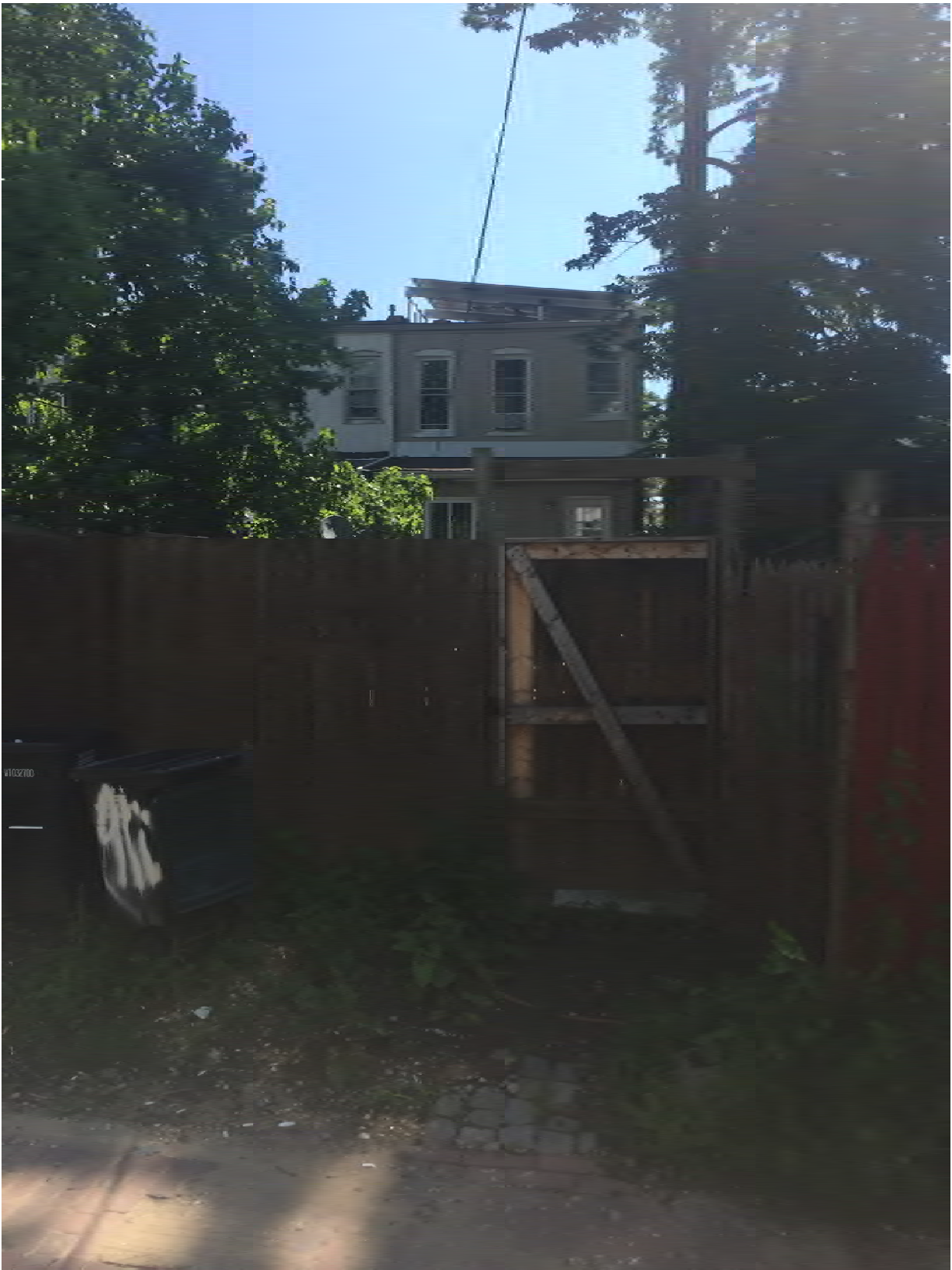
EXISTING YARD FROM ALLEY
