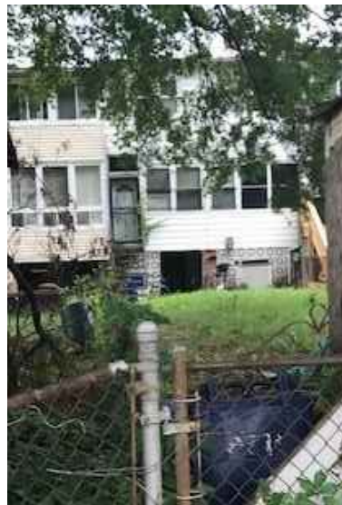
2. VIEW OF EXISTING REAR FACADE
