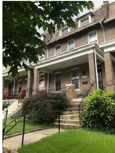
1. VIEW OF EXISTING FRONT FACADE
