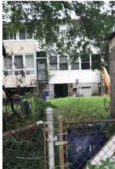
2. VIEW OF EXISTING REAR FACADE
