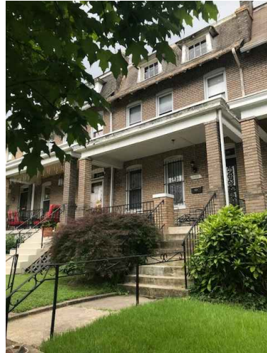
1. VIEW OF EXISTING FRONT FACADE
