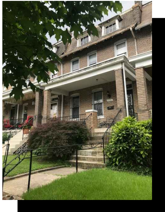
VIEW OF FRONT FACADE
