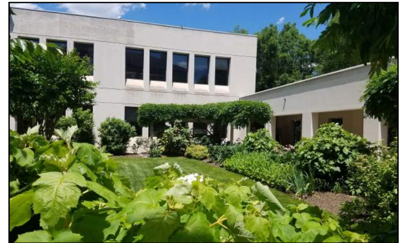
Fig. 1.3.2 - Existing Garden Facade of Chancery
