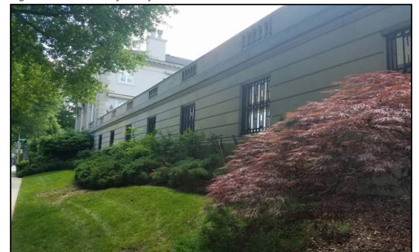
Fig. 1.1.3 - Existing Garden wall and Residence
