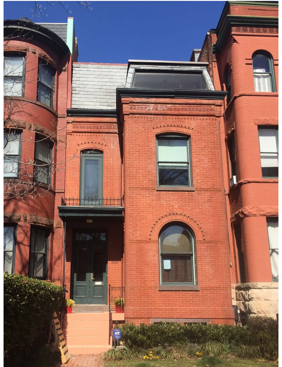
EXISTING FRONT FAÇADE
