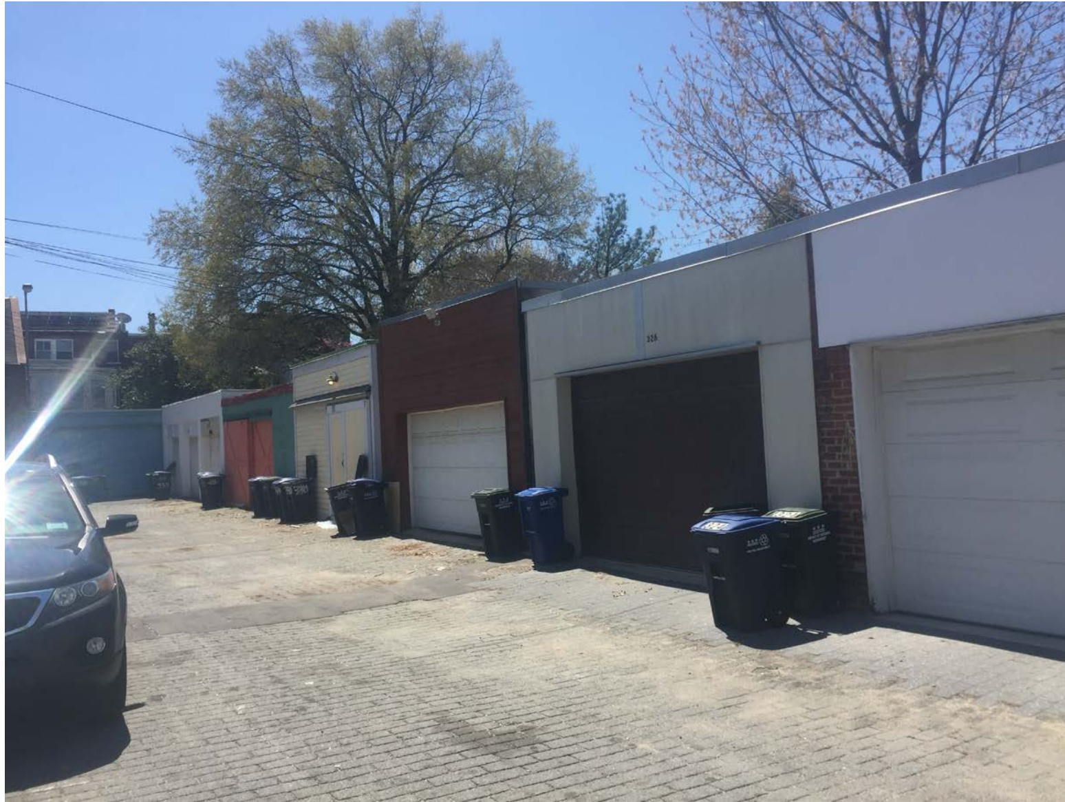
REAR ALLEY LOOKING SOUTH
