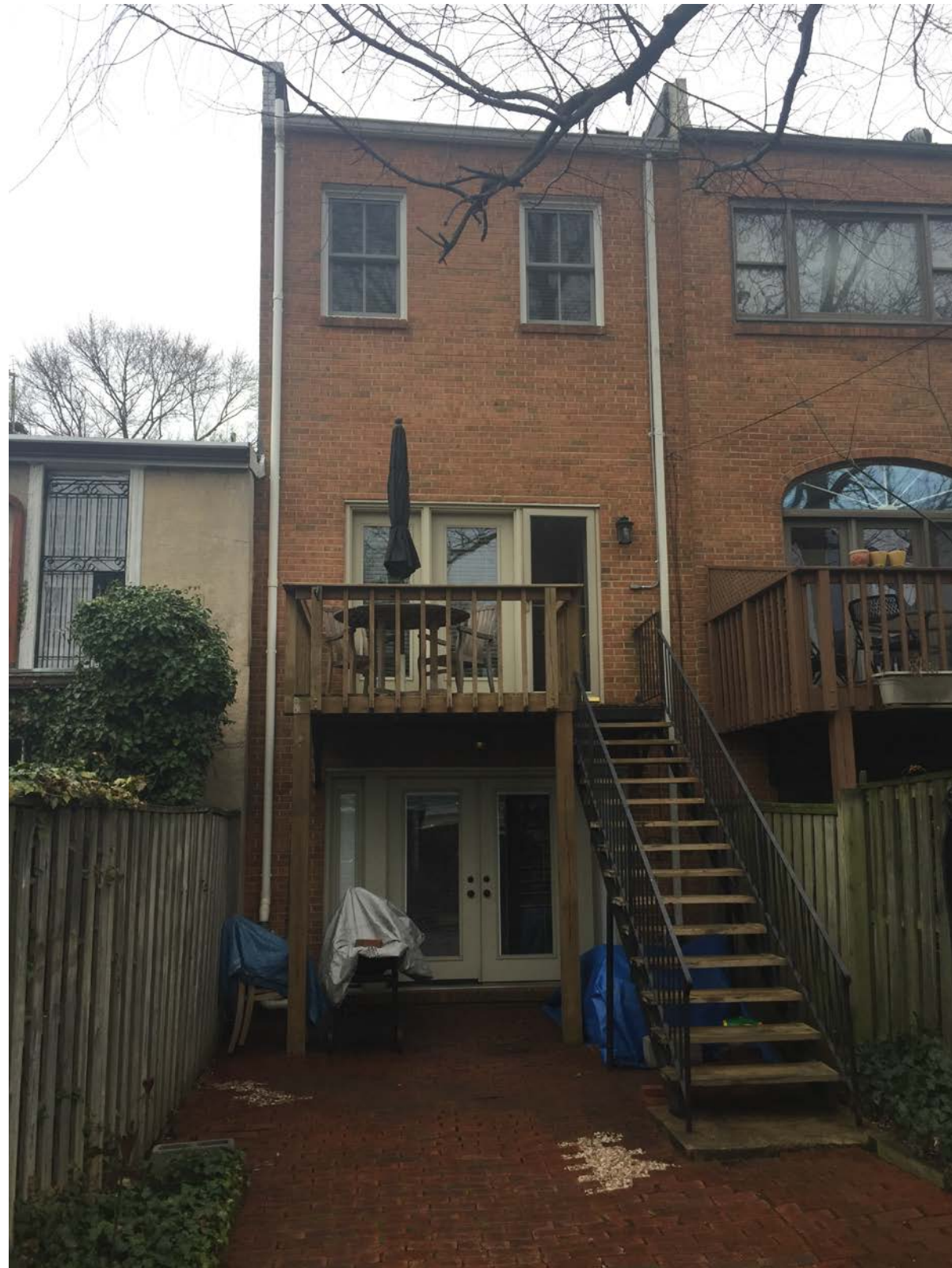
EXISTING REAR FAÇADE
