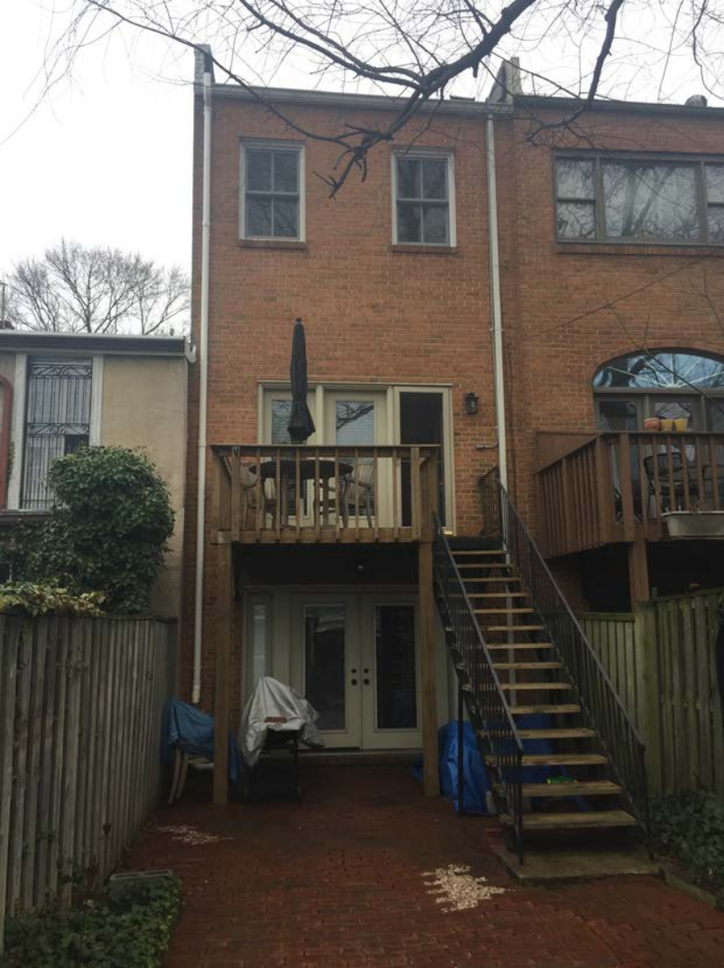
REAR OF HOUSE FROM YARD
