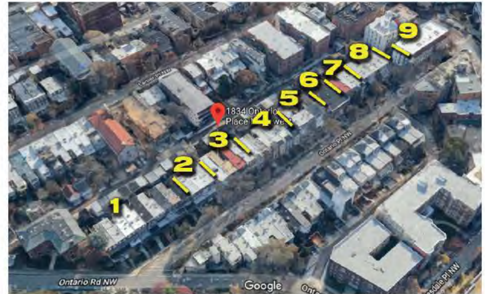
Overview of Block
