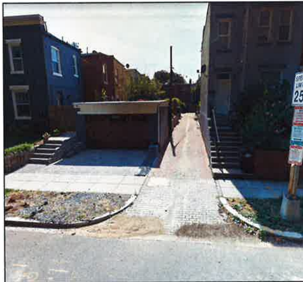
Figure 1 – 445 15th Street SE Accessory Structure (Source: Google Map Streetview, dated June 2017)
