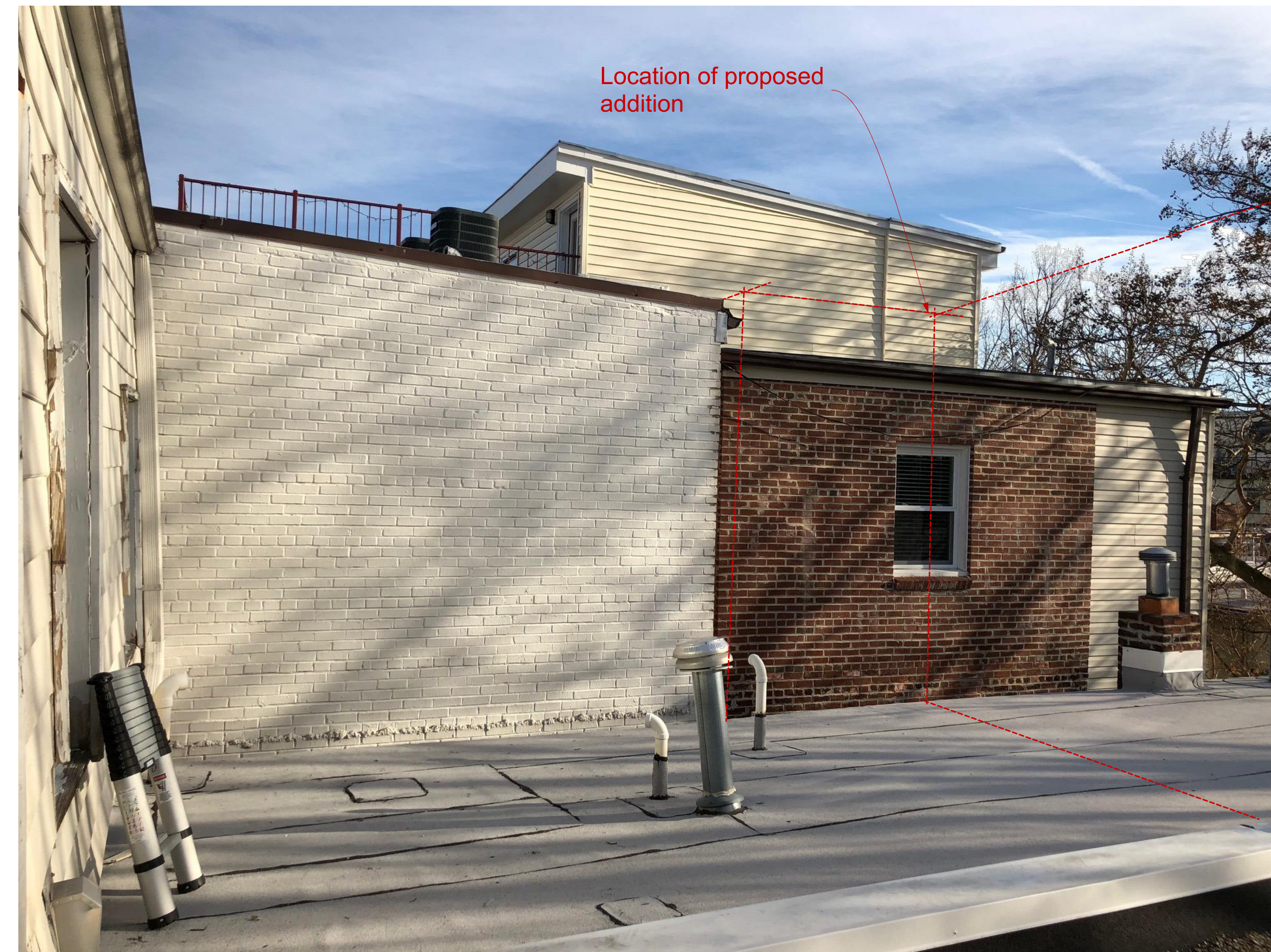
View of 1432 Rear Looking East
