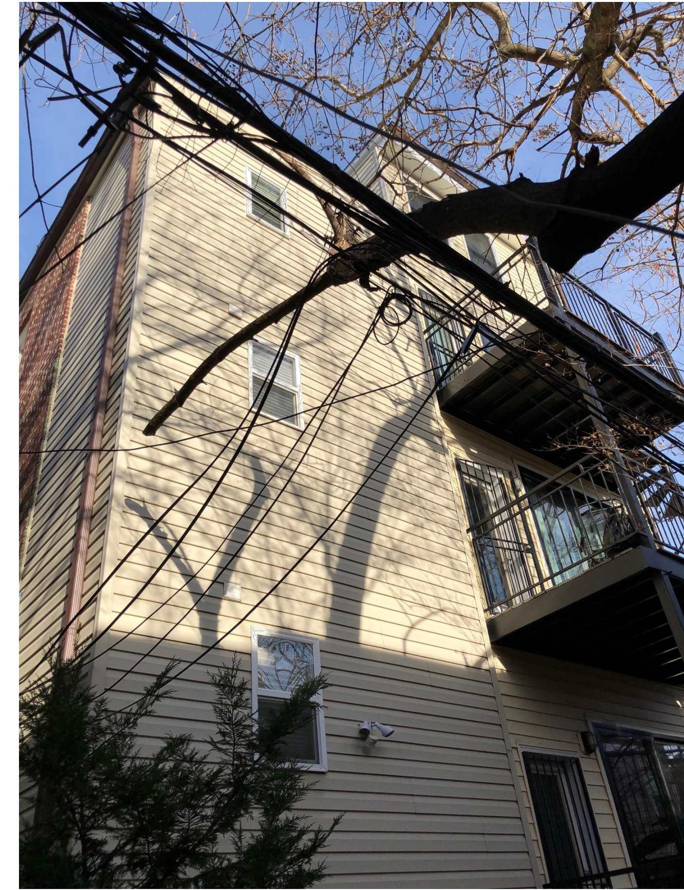
View of 1434 Rear
