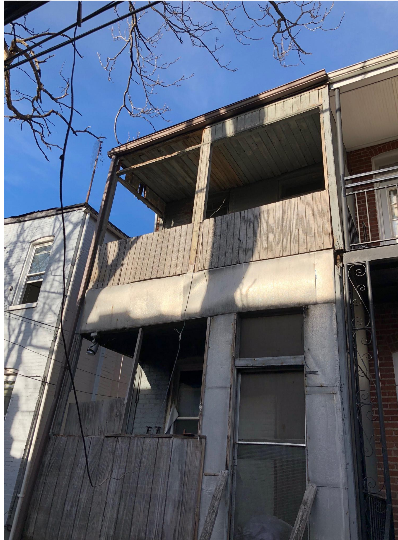
View of 1434 Rear
