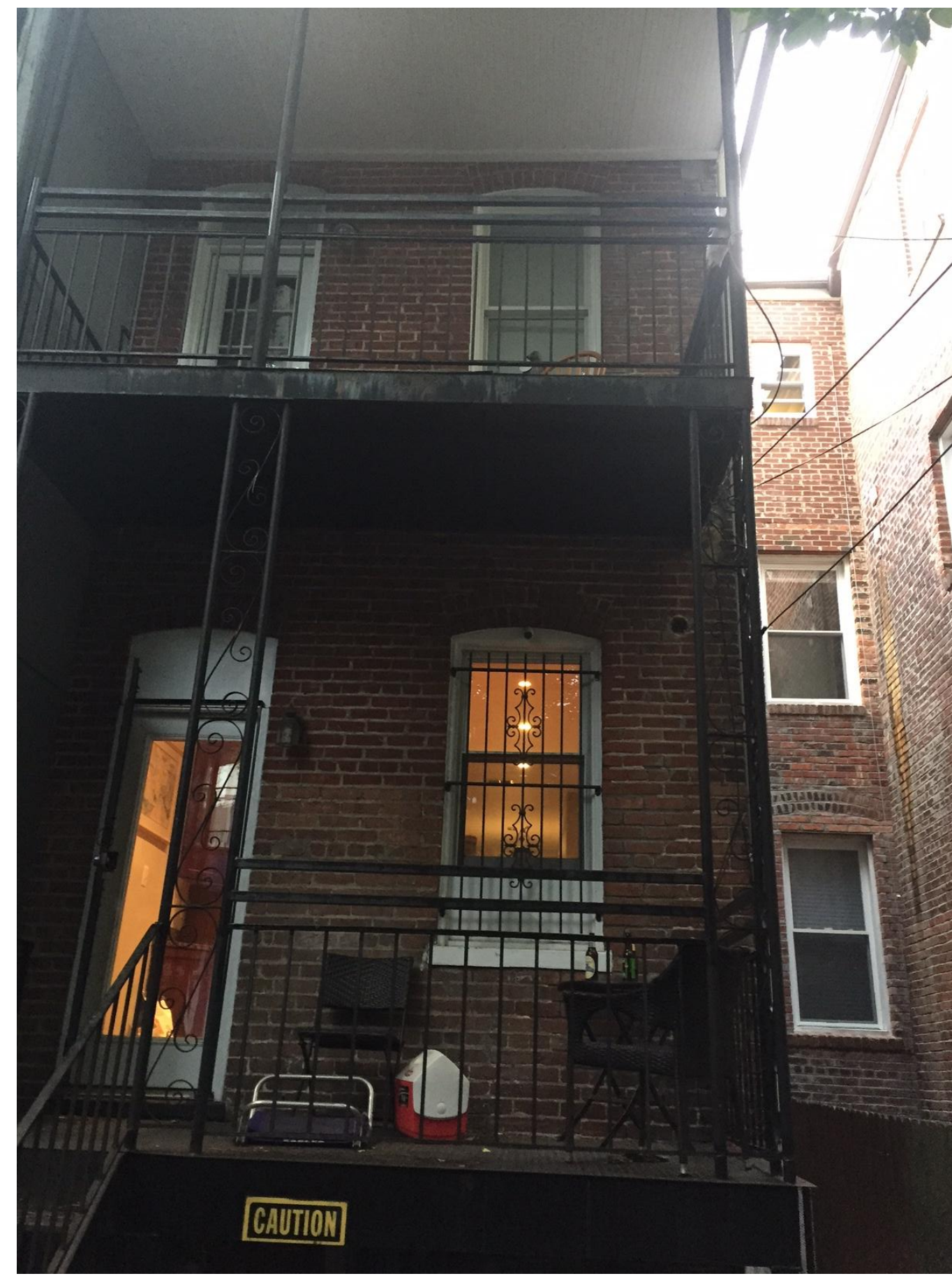
View of 1432 Rear
