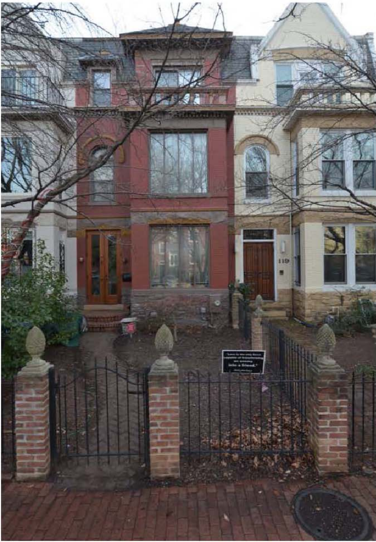
121 TENNESSEE AVENUE NE - EXISTING FRONT FACADE
