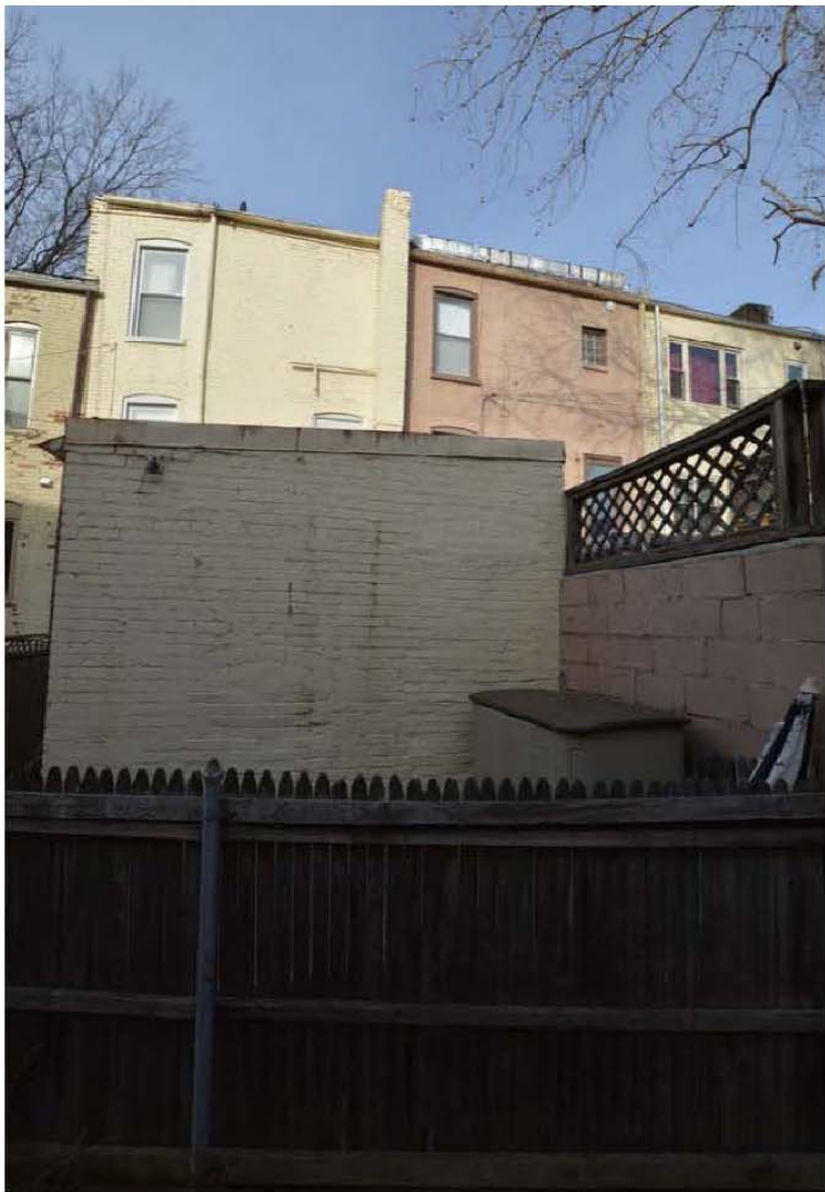
119 TENNESSEE AVENUE NE - NEIGHBOR TO THE SOUTH
