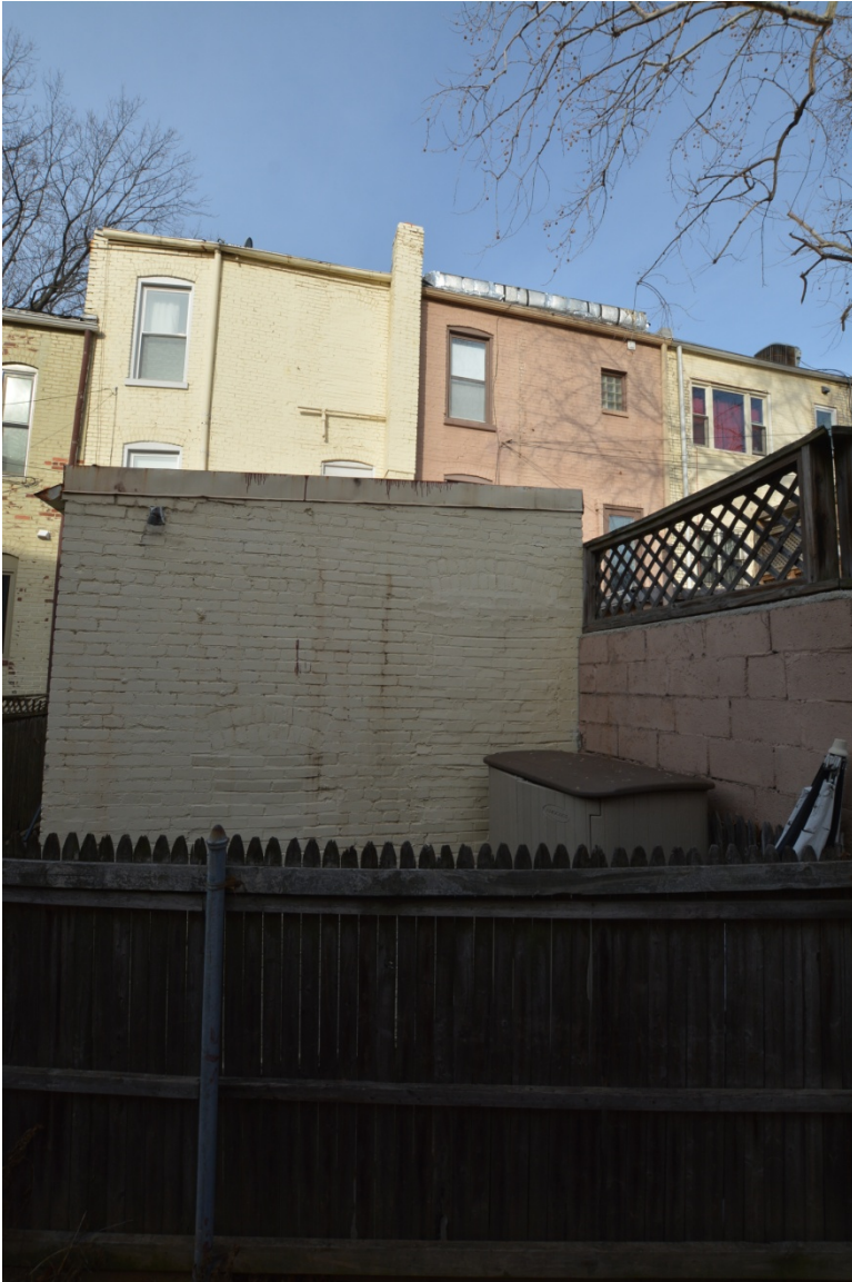
119 Tennessee Ave NE (Rear), Neighbor to the South
