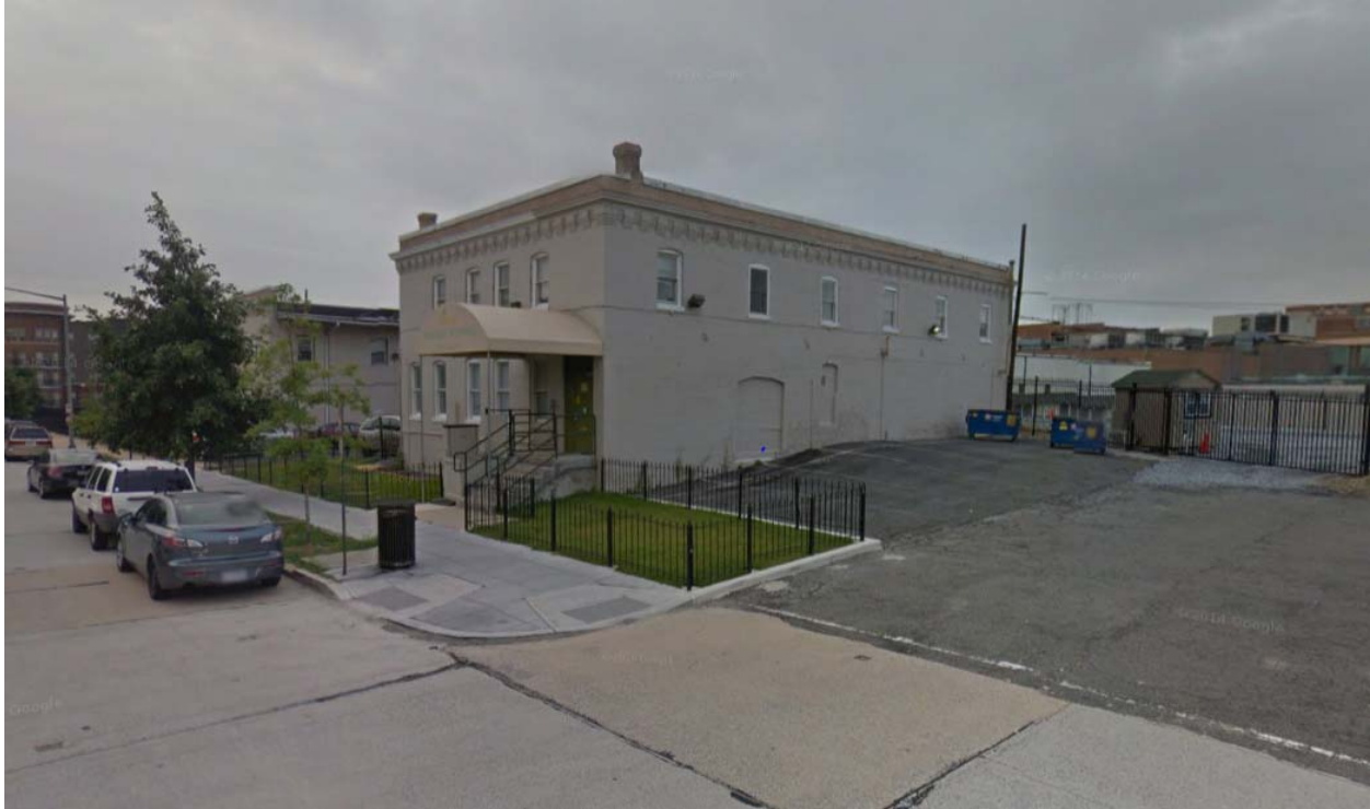
From the northwest corner of the property looking southeast
