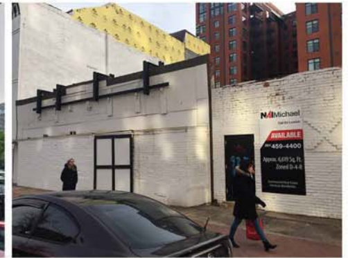
EXISTING BRICK FACADES
