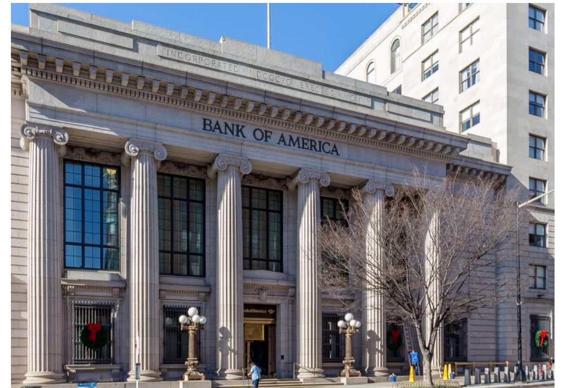
D. From Corner of New York Ave. and 15th Street Looking Northwest
