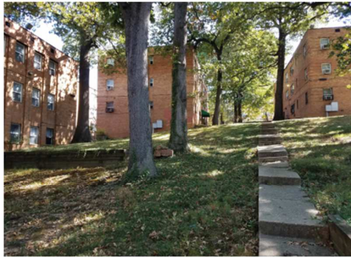
6. Existing interior open space looking east
