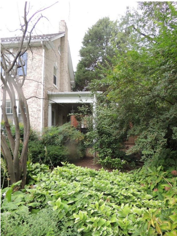
View of the East (Reno Road NW) Elevation with the porch
