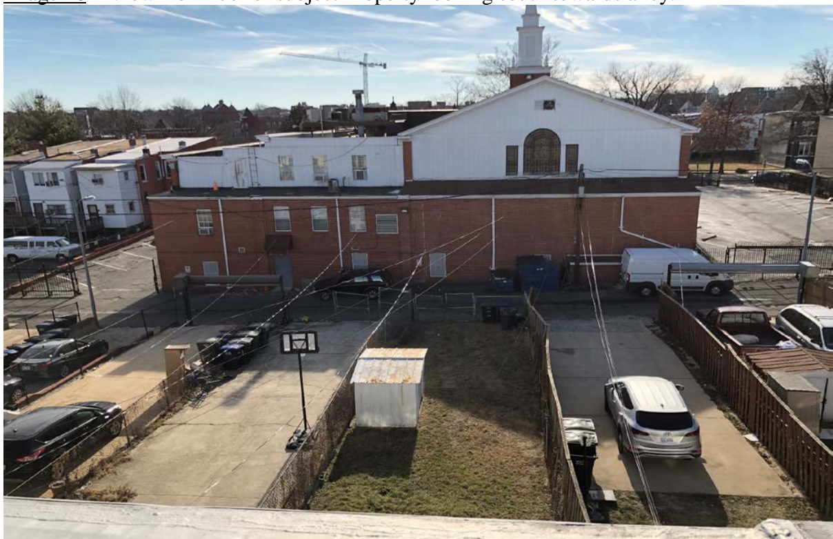
Image #6 – View from roof of subject Property looking south towards alley.
