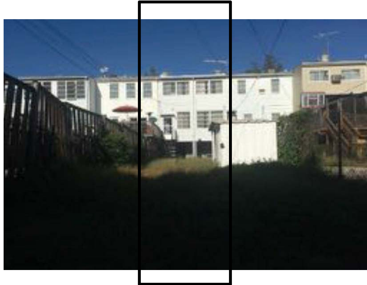
1135 MORSE ST. NE REAR FACADE
