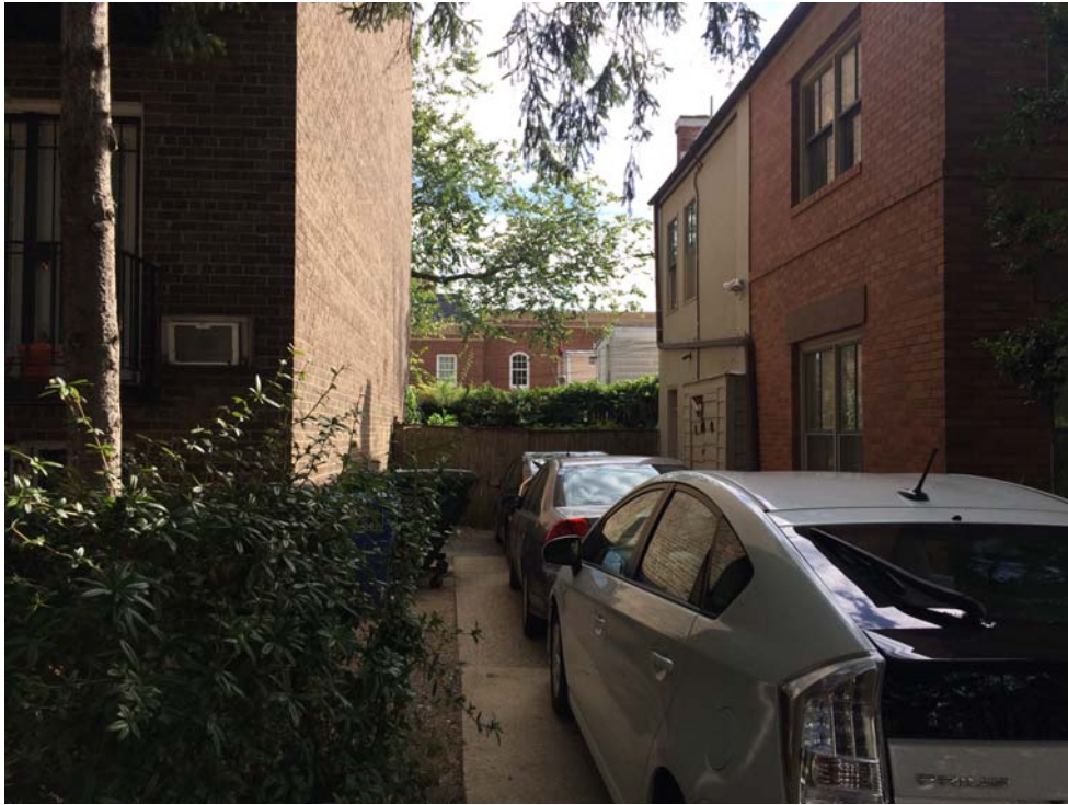
View from E Street SE through rear yards
