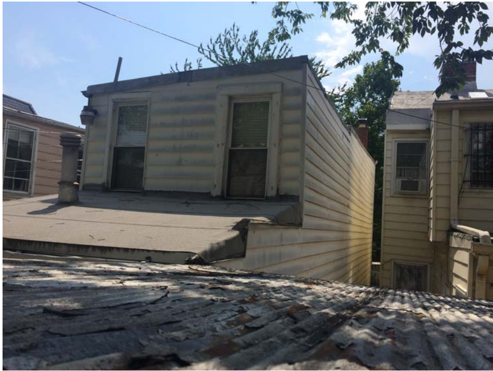
View of north façade from rear
