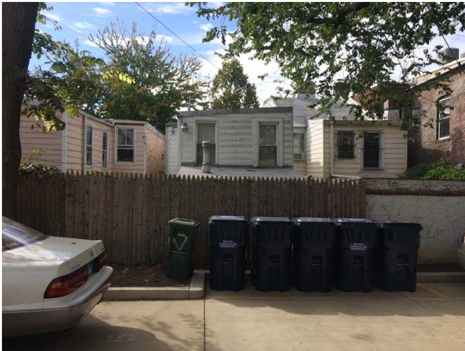
View of 1506 E Street SE from rear yard
