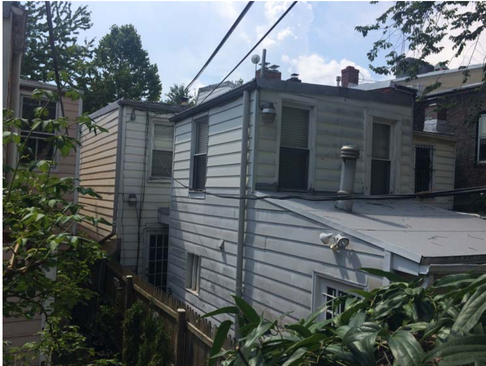
View of south façade from rear
