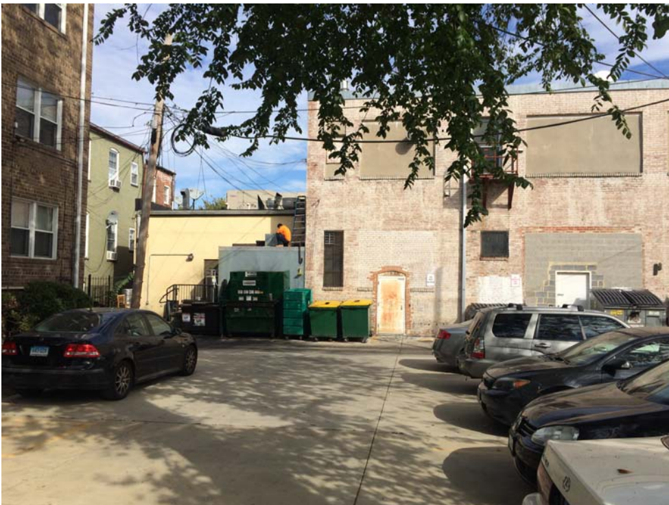
View from rear yard towards alley
