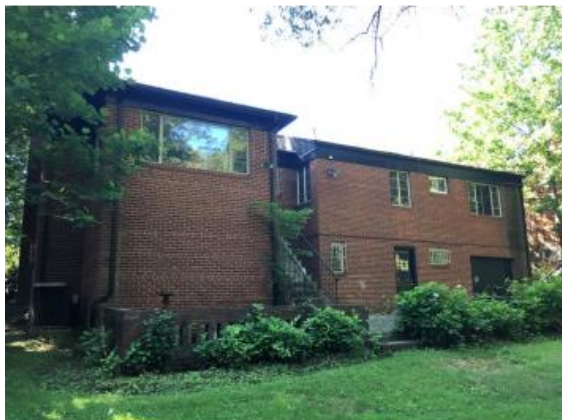
Rear of House
