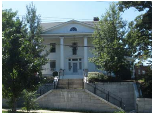
DC DREAM CENTER - 2909 PENNSYLVANIA AVE, SE 2 STORIES
