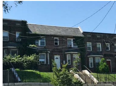
RESIDENCES - 2915-2923 PENNSYLVANIA AVE, SE 2 STORIES
