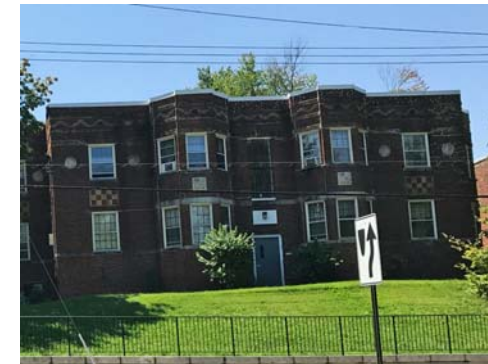
RESIDENCES - 2925-2929 PENNSYLVANIA AVE, SE 3 STORIES
