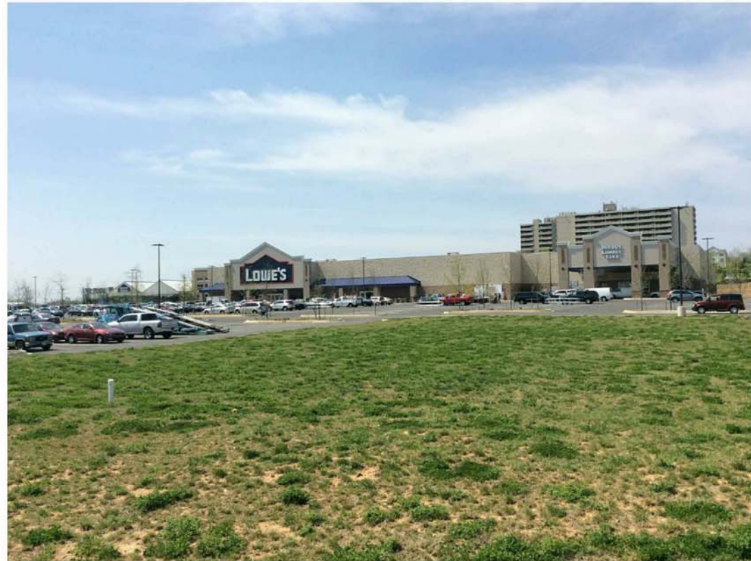
PHOTO 3 - VIEW OF EXISTING PROPERTY FACING EXISTING LOWE'S.
