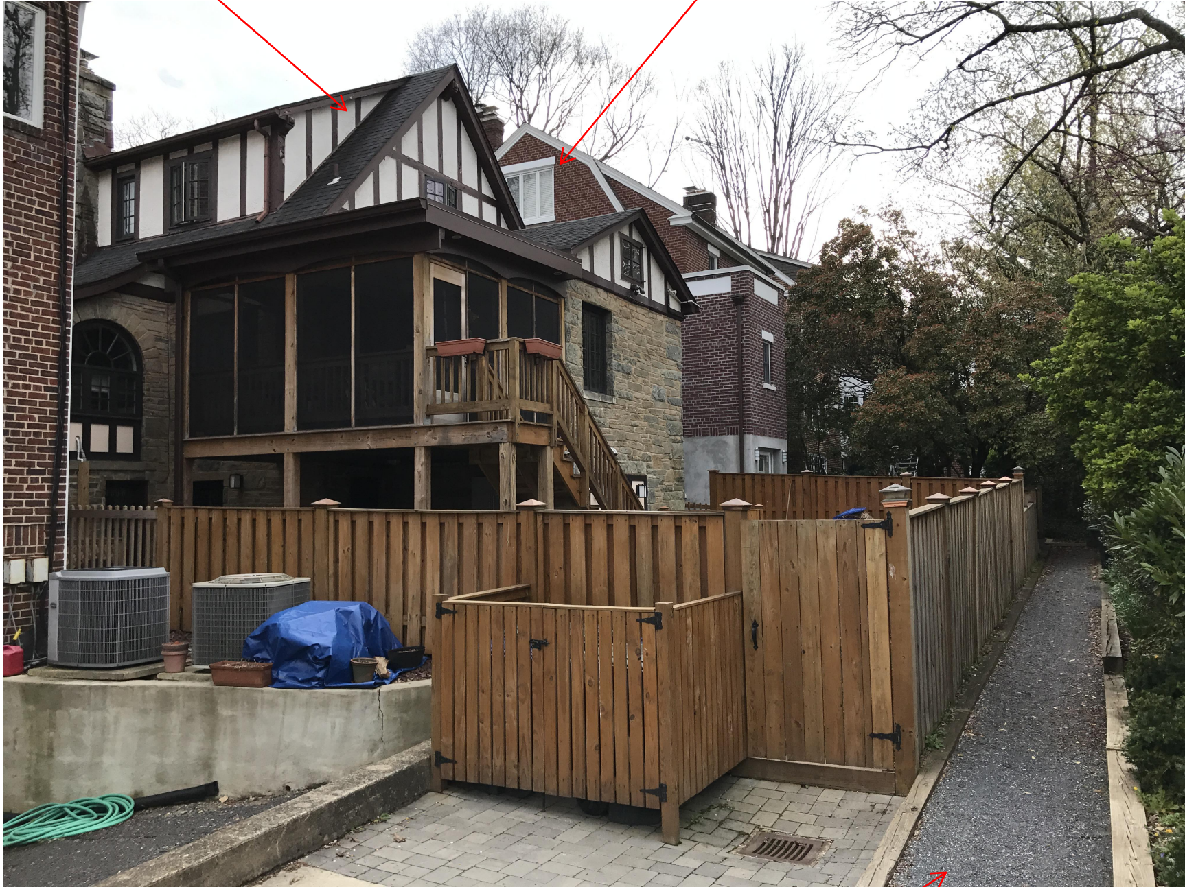
PHOTOGRAPH - REAR YARD FROM REAR ALLEY
