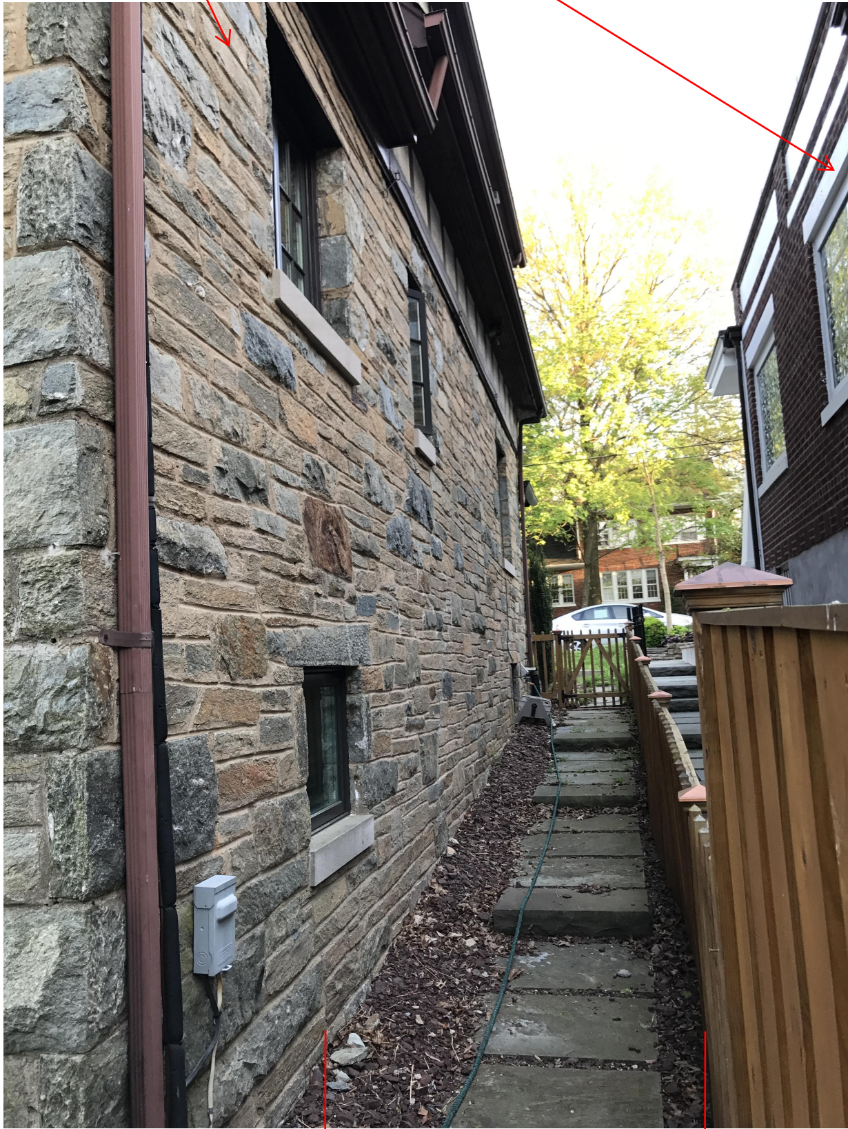
PHOTOGRAPH - WEST SIDE YARD FROM REAR YARD
