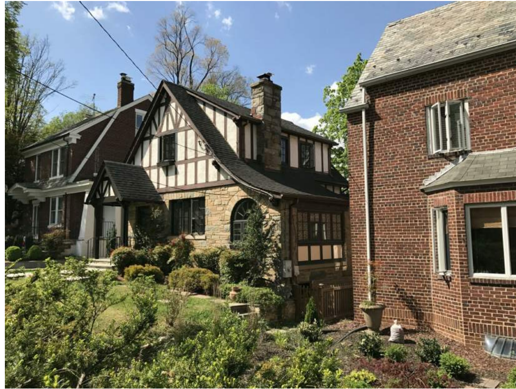
① PHOTO - FRONT YARD FROM PATTERSON ST NW 12" = 1'-0"
