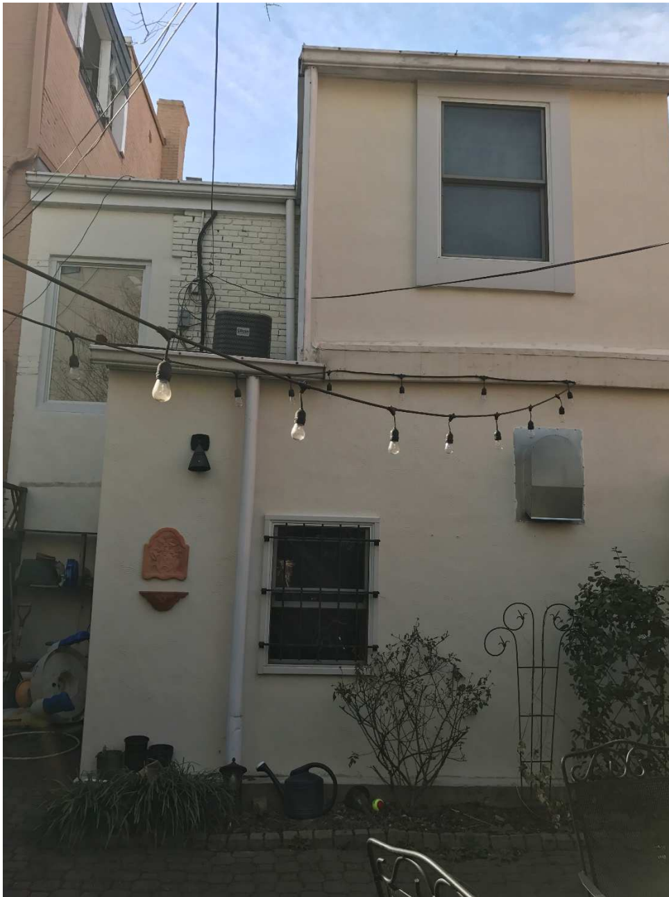
Image #4: Rear view of 1519 12 th Street, NW
