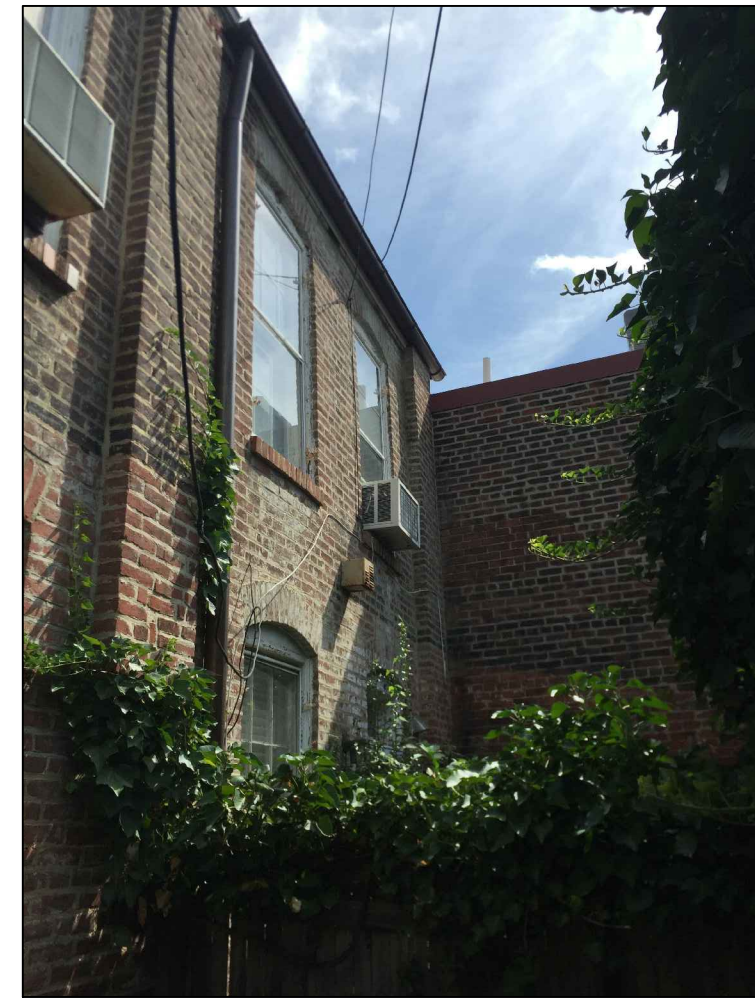
REAR (SOUTH) FACADE
