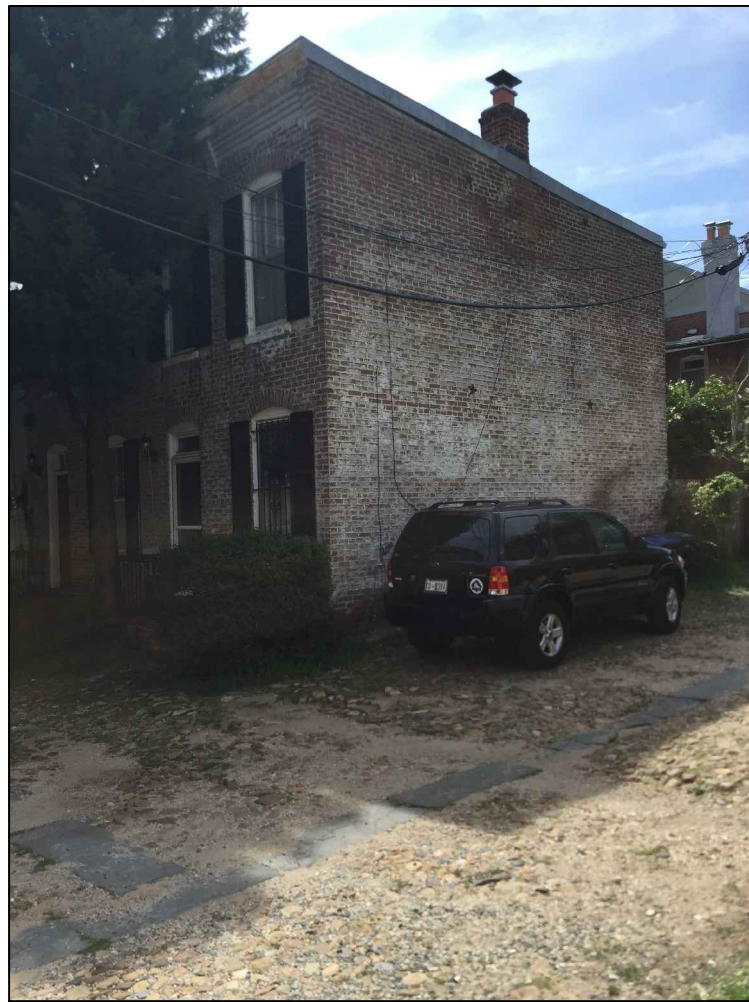
FRONT (NORTH) AND SIDE (WEST) FACADE
